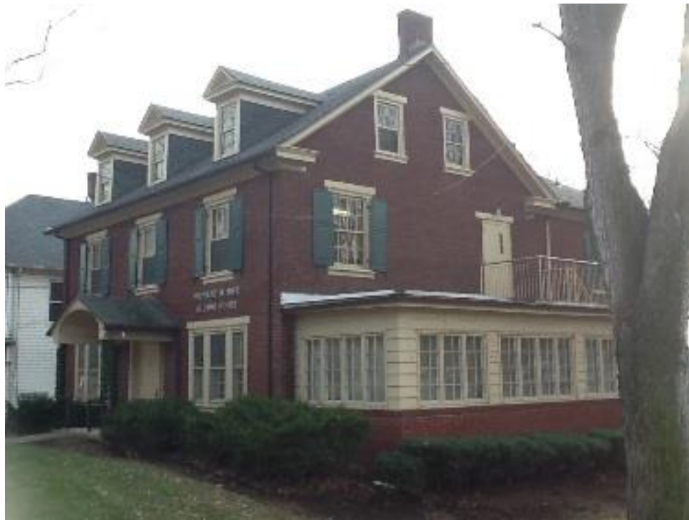
Shippensburg University Rife Alumni House; right-front elevation. (Image by Michael D. Griesemer)
