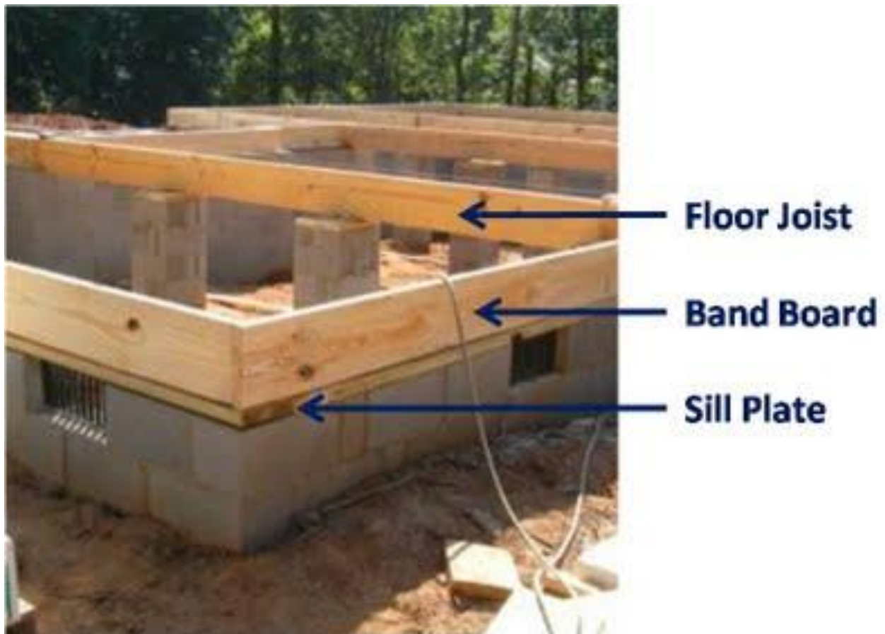
Figure 2: Basement Rim and Band
