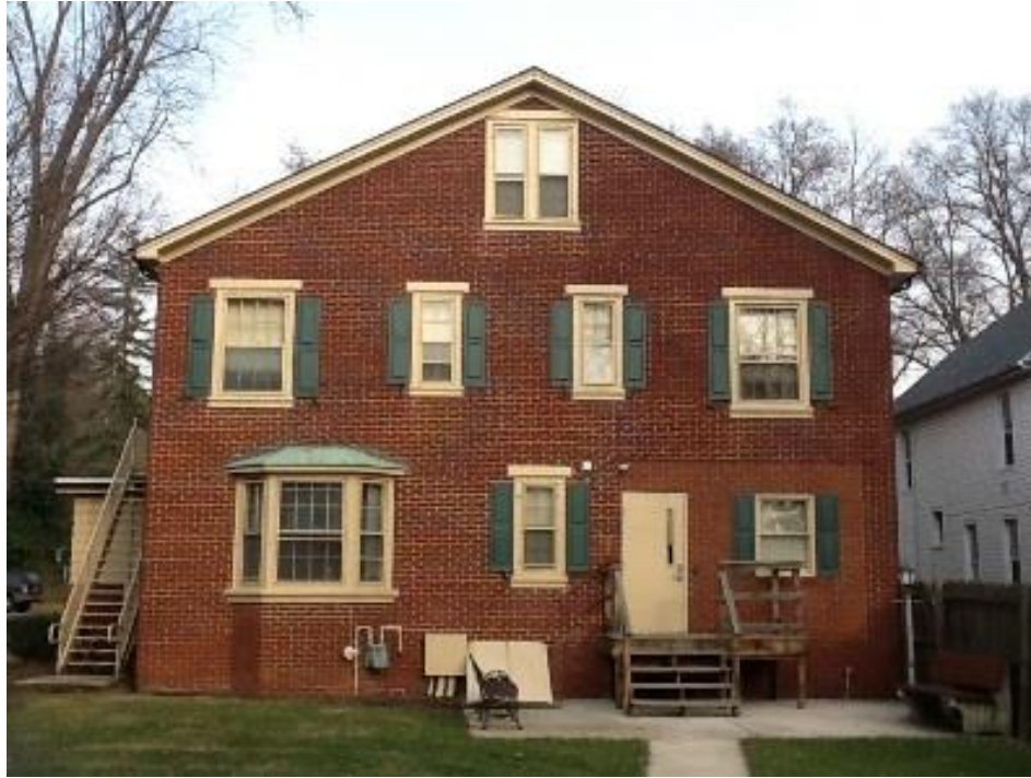
Shippensburg University Rife Alumni House; rear elevation. (Image by Michael D. Griesemer)
