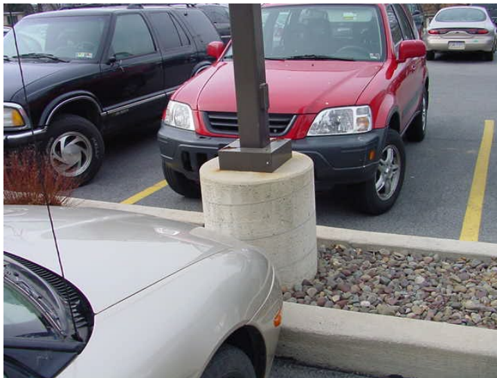
Protected base at Gilbert Lot
