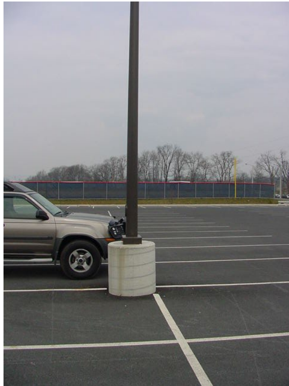
PAC Commuter Lot Lighting Base
