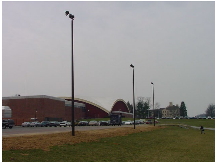
Direct Bury Pole for Parking Lot Lighting
